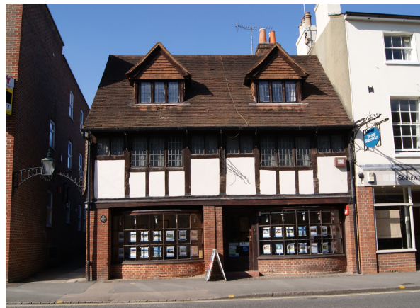
West Street, Farnham: The use of a brick for the stall riser respects the character of the building. The stall riser is proportionate to the building and elevates the window to eye level.
